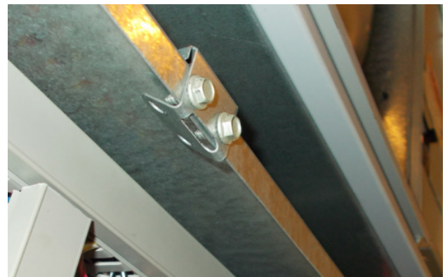
FIGURE 8 Re-Install Screws and Bend Tabs Up
