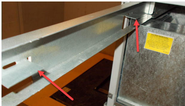
FIGURE 4 Filter Tabs in Up Position
