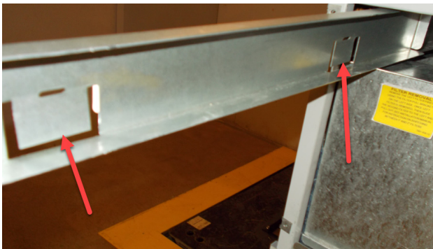
FIGURE 5 Bend Filter Tabs Down
