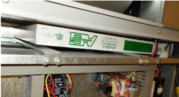
FIGURE 10 Install Left 2" Filter
