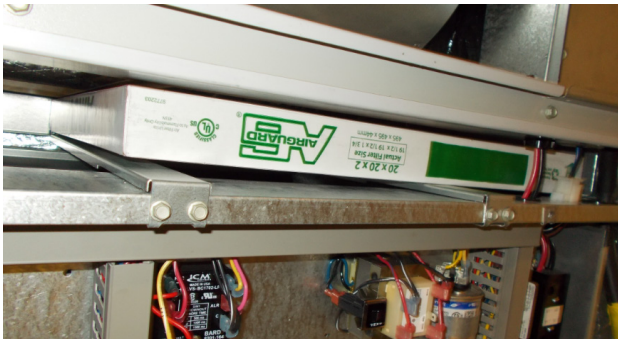
FIGURE 10 Install Left 2" Filter
