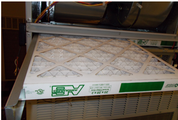
FIGURE 10 Install Left 2" Filter
