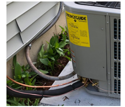
Install Linesets and Electrical
